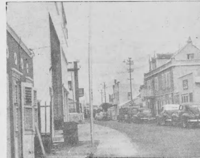
at the right, looking west, shows excellent sidewalks, a paved road, and the new building of the Aruba Commercial Bank (left side of street). Note the network of power and telephone lines in the new picture.
